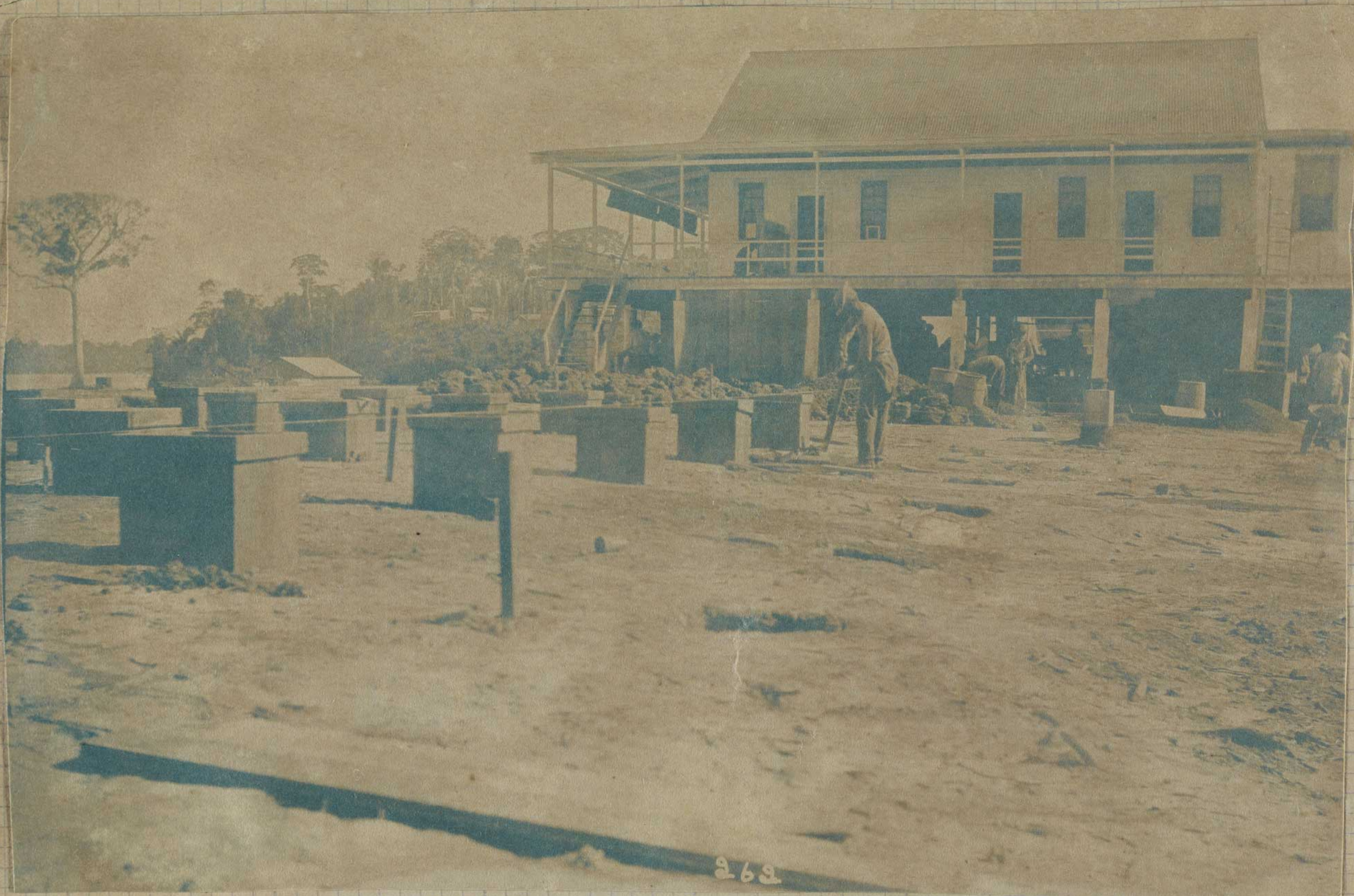
Foundation for Engineer's quarters
