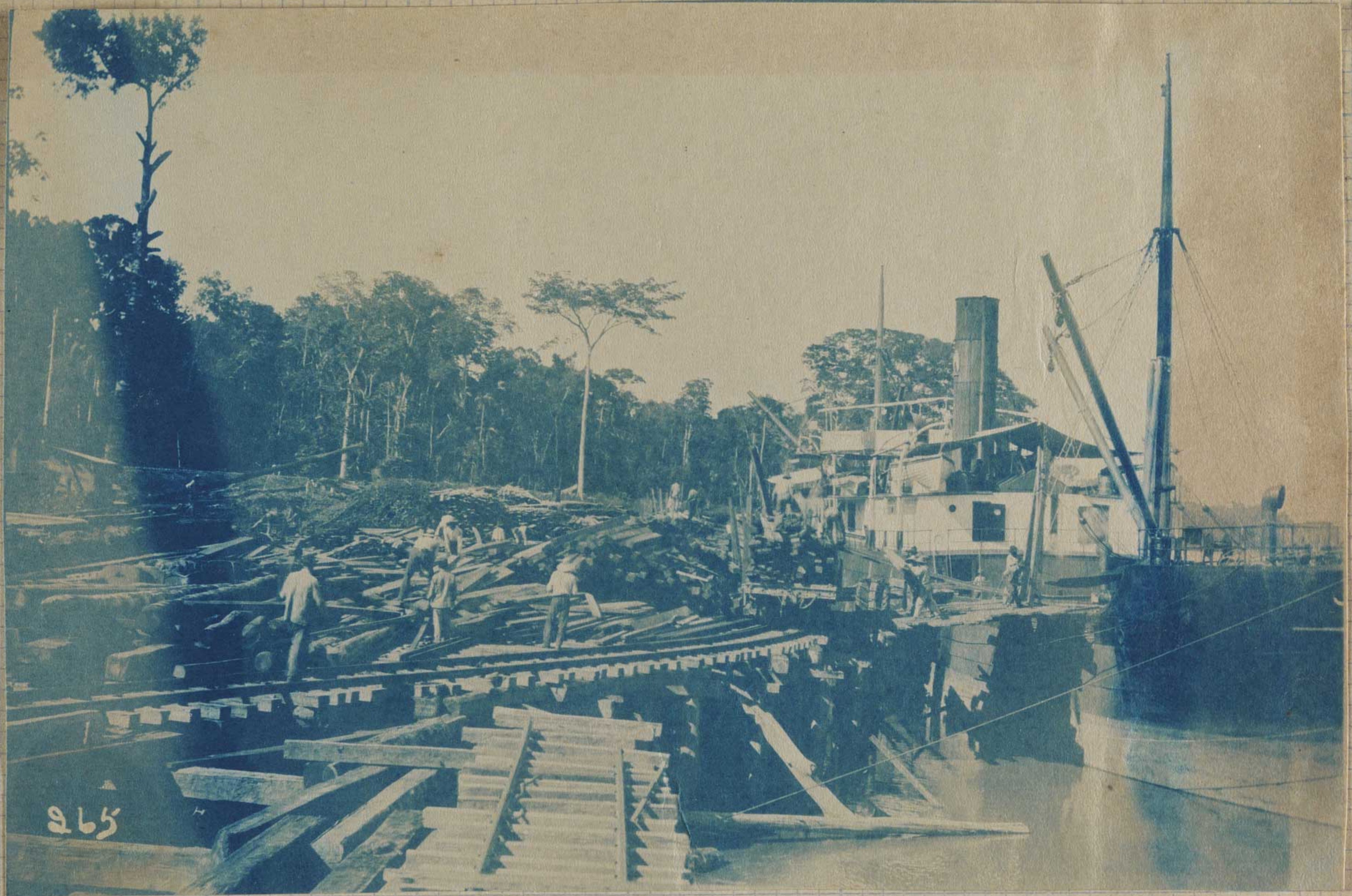
Unfinished Wharf, and "Steam Ship Falk"
